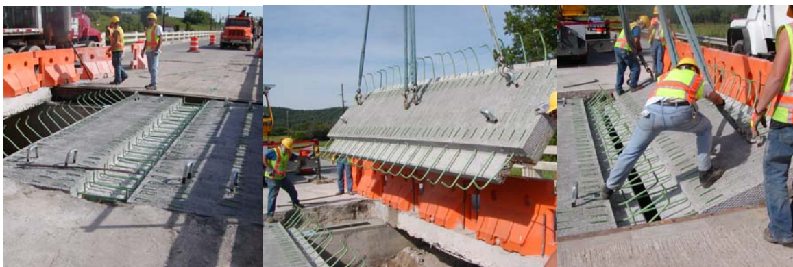
Figure 9 Maintenance crews retrofitting Bridge 6679 with PCSSS panels
